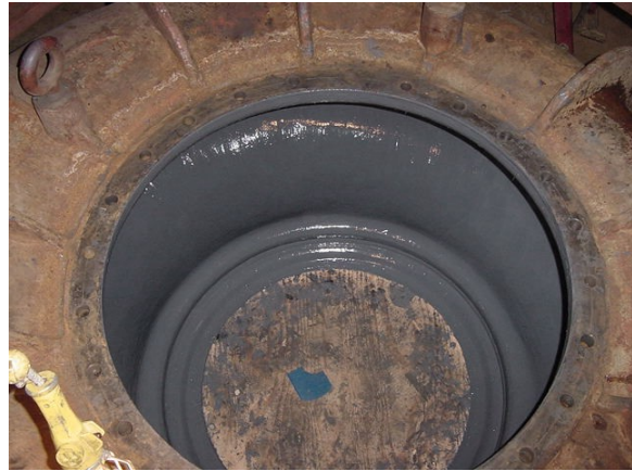
ARC 855 coating system installed
