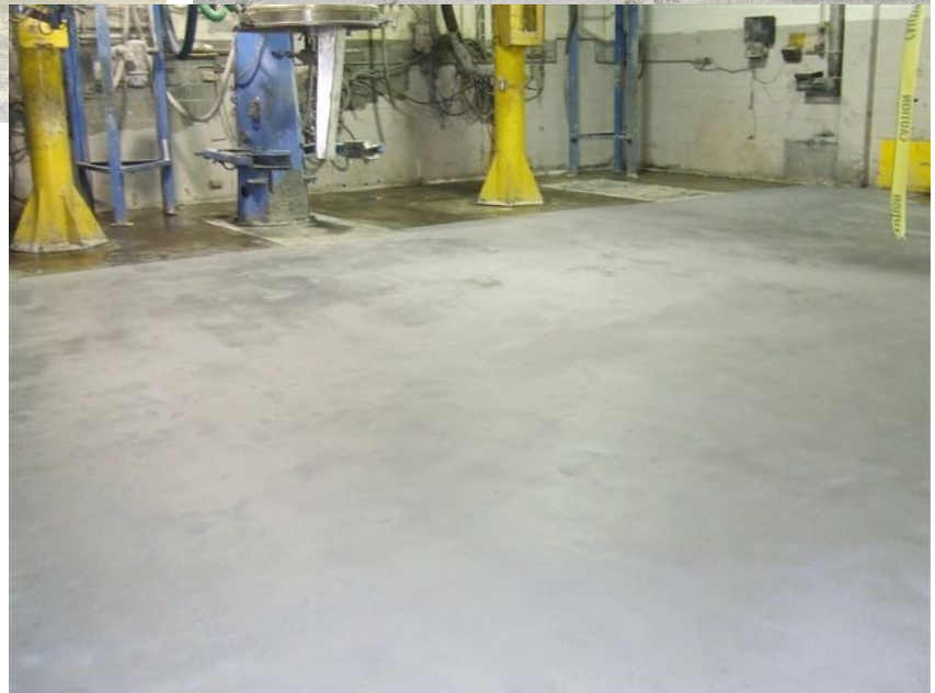
Right – Area leveled, 3300GS Installed, awaiting 1000CS Topcoat.
