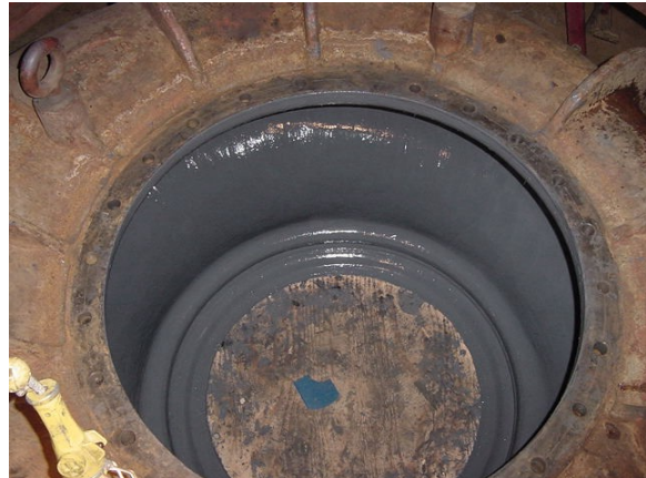
ARC 855 coating system installed
